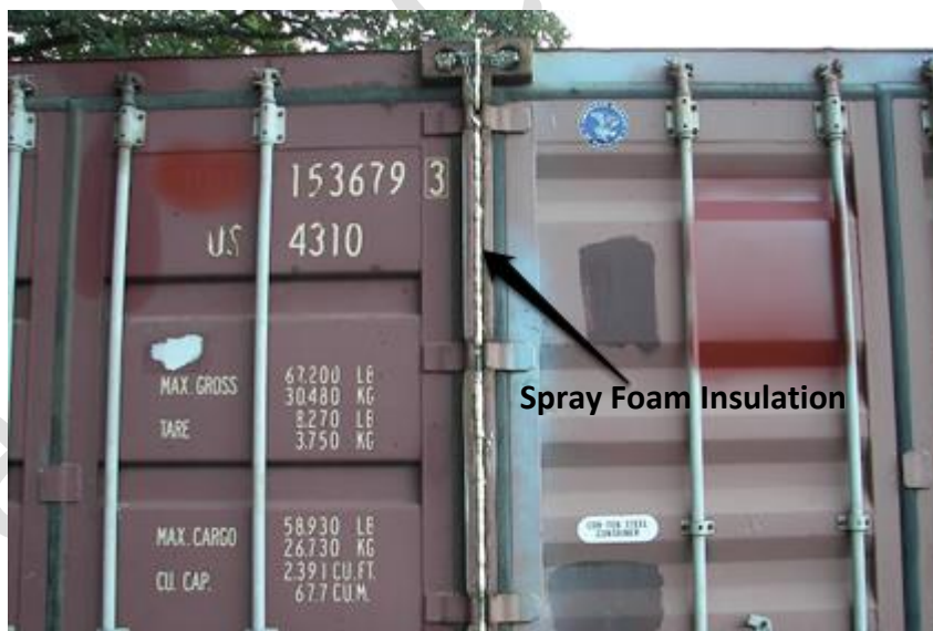
Figure 8.5: Insulating Shipping Container
