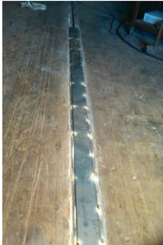
Figure 8.10: Welding Shipping Container Floor
