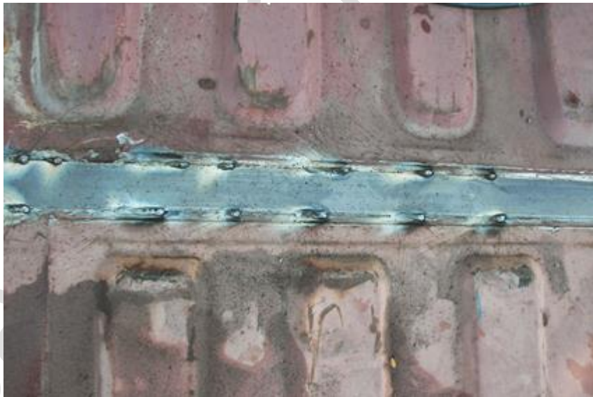
Figure 8.7: Welding Shipping Container Roof
