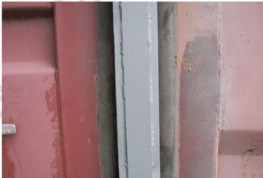
Figure 8.9: Welding Ends Of Shipping Container
