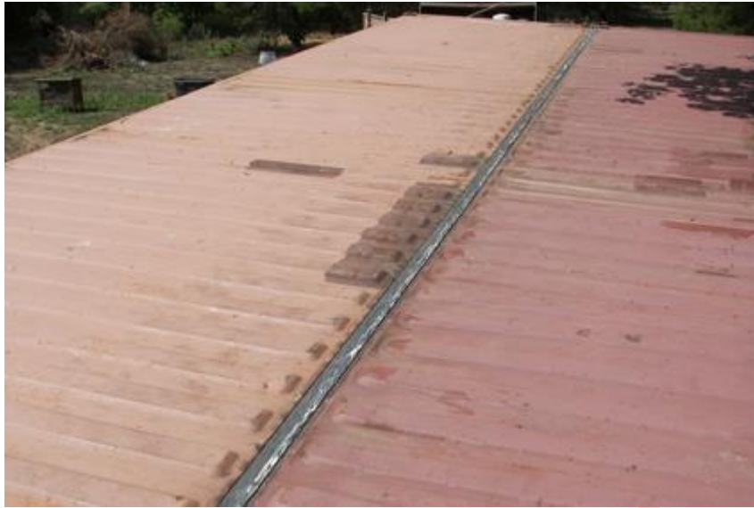
Figure 8.8: Finished Welding Shipping Container Roof
