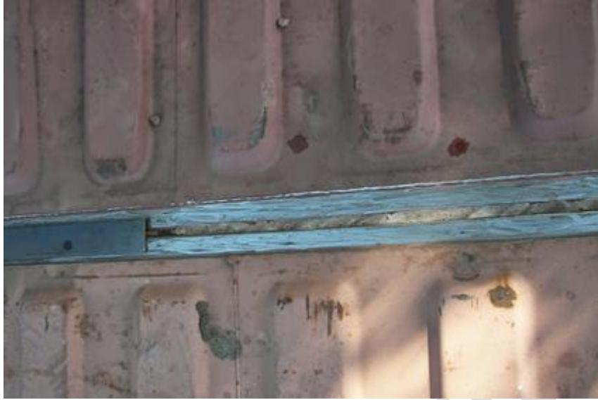
Figure 8.6: Welding Shipping Container Roof
